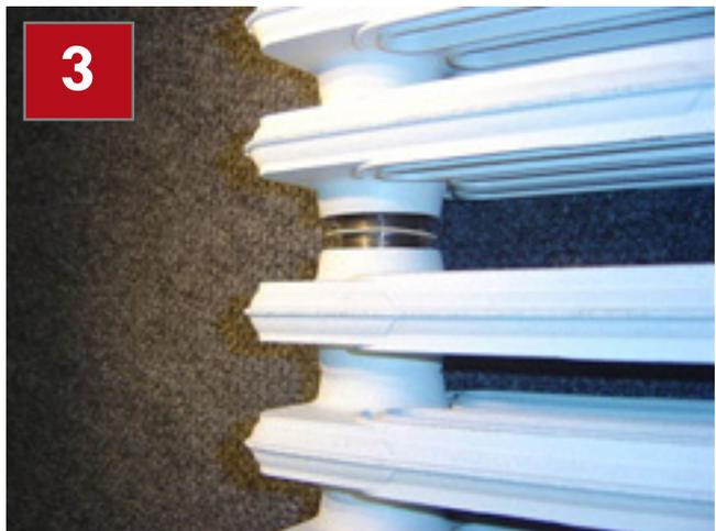
Carefully slide the second section next to these nipples, taking care that the thread connections are correct.
