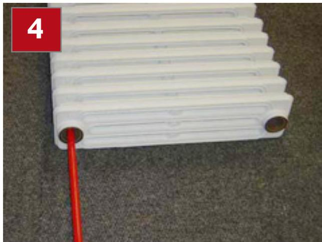
Rotate the nipple using the nipple key, so that it pulls the 2 sections together. At this stage only rotate the nipple by one turn. Repeat with the other nipple.
