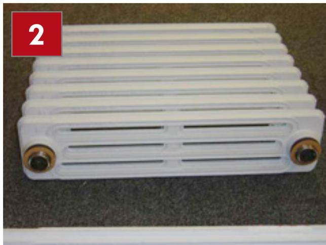
Screw a pair of nipples into one end of the radiator. Only screw in by one turn, do NOT screw in fully. Place a gasket approximately at the mid-point of each nipple.
